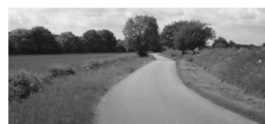
Fig. 3. Narrow roads constrain movement of wide vehicles
